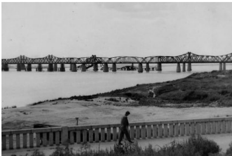
Figure 128: Damaged Han River Bridge
