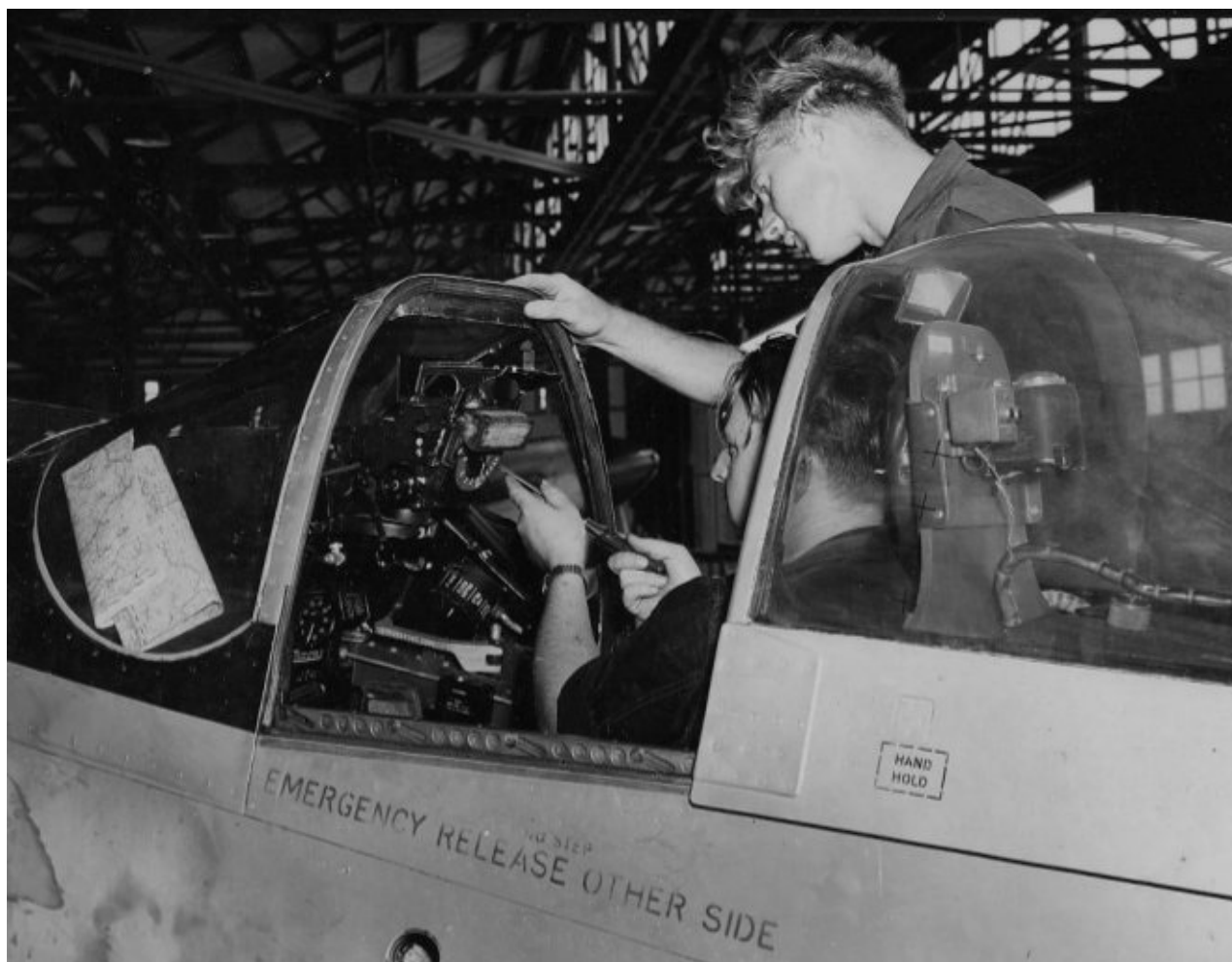
Figure 81: Adjusting Mustang Gyroscopic Gunsight
