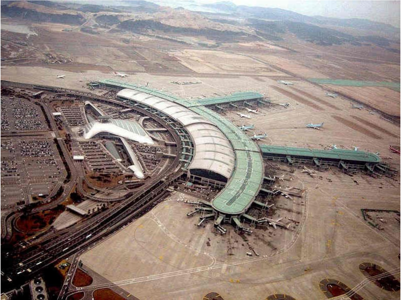
Figure 206: Incheon International Airport
